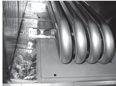
Figure 17: Discharge panel in place
